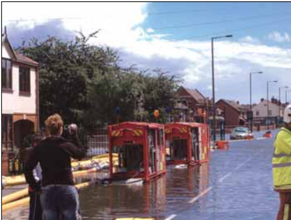
The High Volume Pumps (HVPs) in use during the recent heavy flooding
