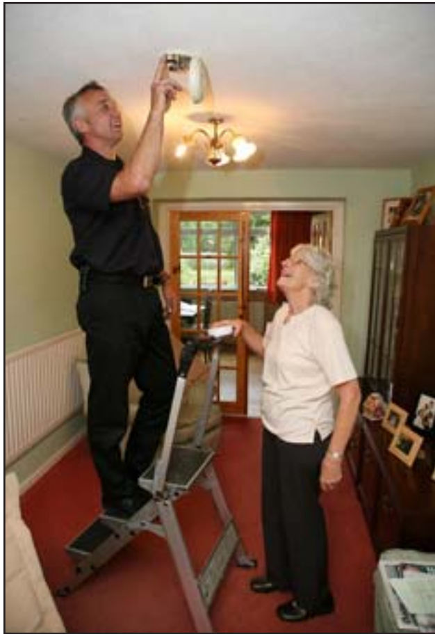
Fitting a smoke detector
