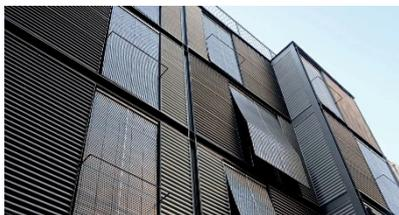
Some buildings such as tower blocks have **cladding** made from **Aluminium Composite Materials**.
