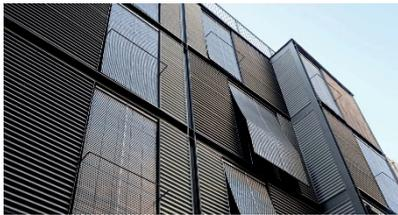
**Aluminium Composite Material** is used to make a type of **cladding**.
