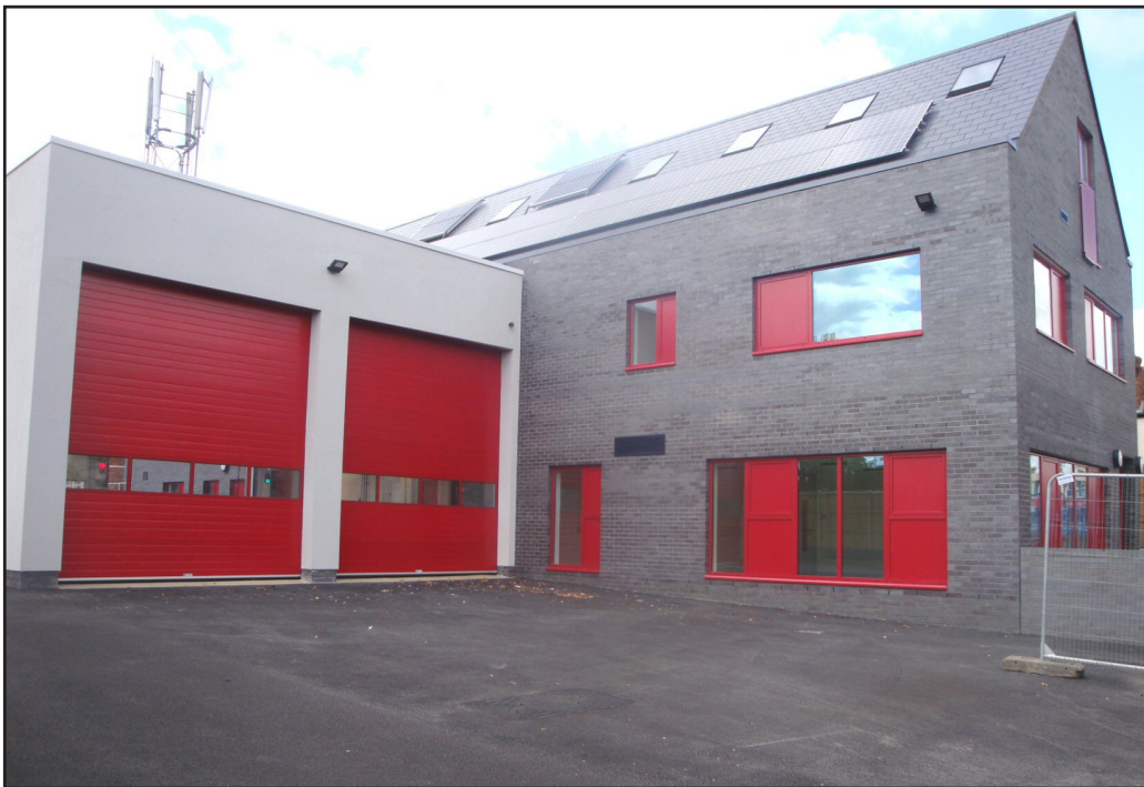
The new fire station at Wokingham
